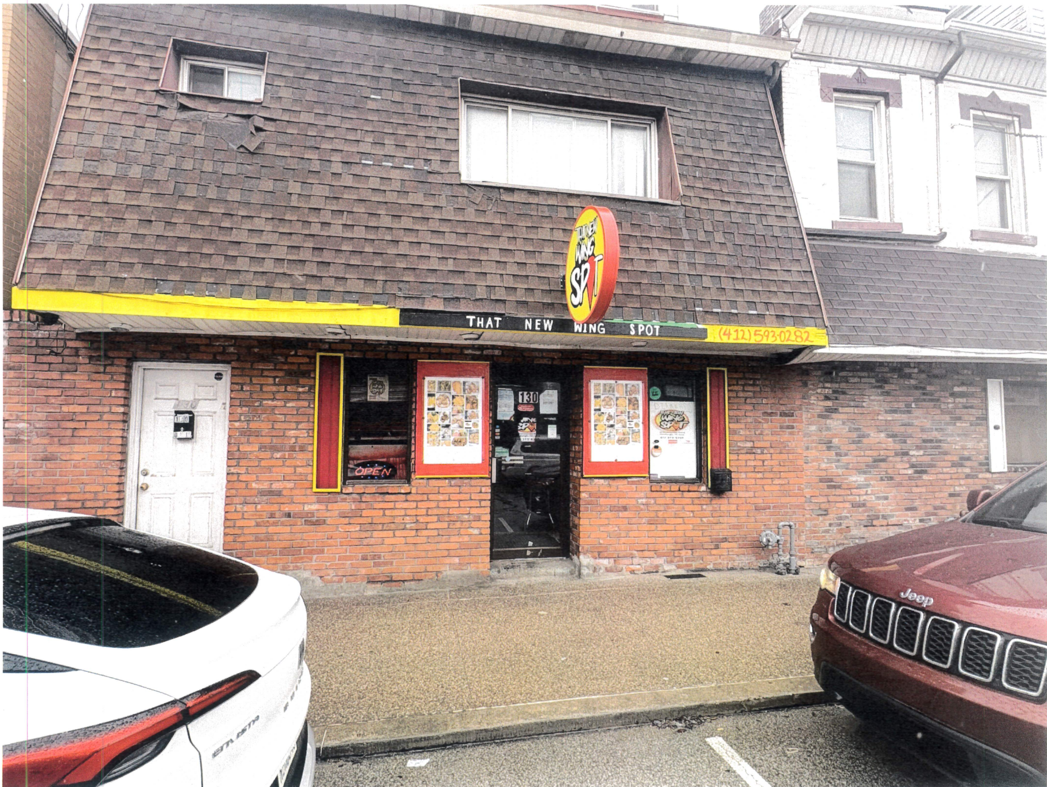
130 Brownsville Existing-condition photograph
